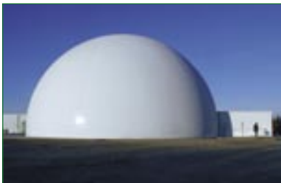
The completed radome.
