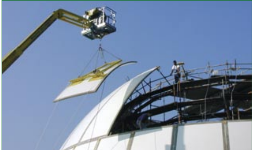
The Divinycell-cored panels being 'slotted' into place to create the radome.
