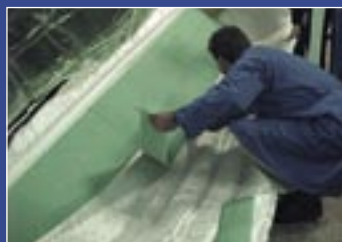
Placing the core.
